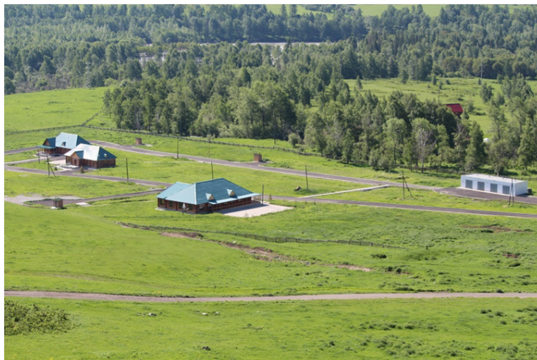
Figure 3 – Administrative and Residential Buildings on the Territory of the Museum Complex
